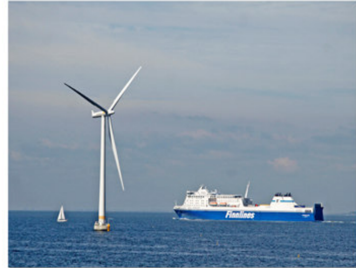
Lilgrund Wind Power Plant, 2009-2010 The first windturbine on Lilgrund.
